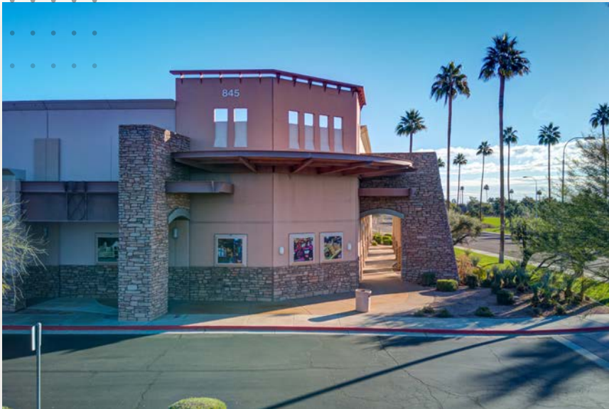
South Side of Subject Facing ICE DEN
